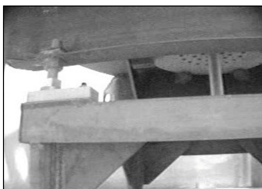
Figure 6. View of the reactor structure.
