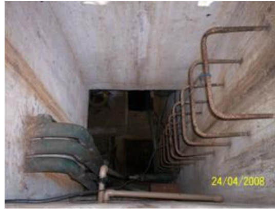
Internal access to effluent retention tank TR1
