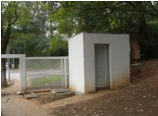
Sewerage discharge point E1 Station
