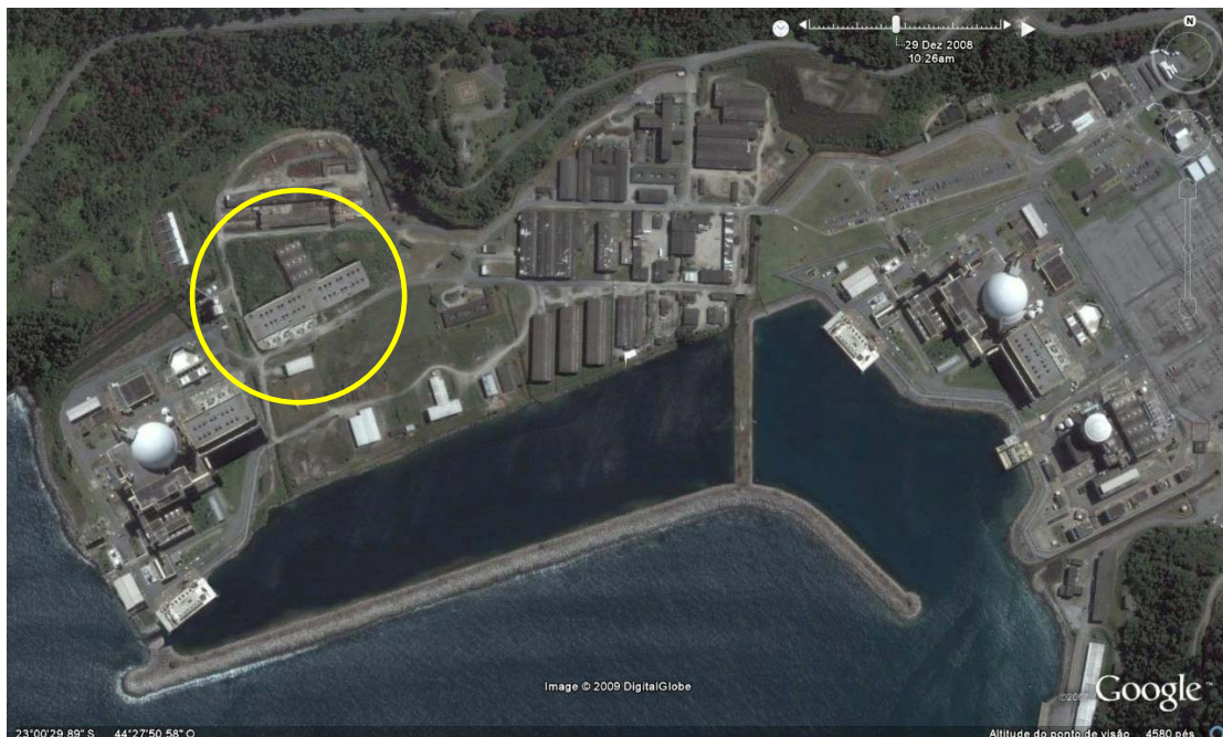
Figure 5. Aerial view of a possible location of SNF dry storage installation at Angra's reactors site.
