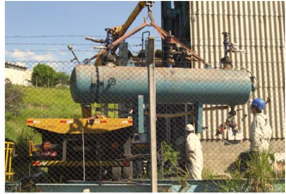
Fig 5 - Secondary crystallizer
