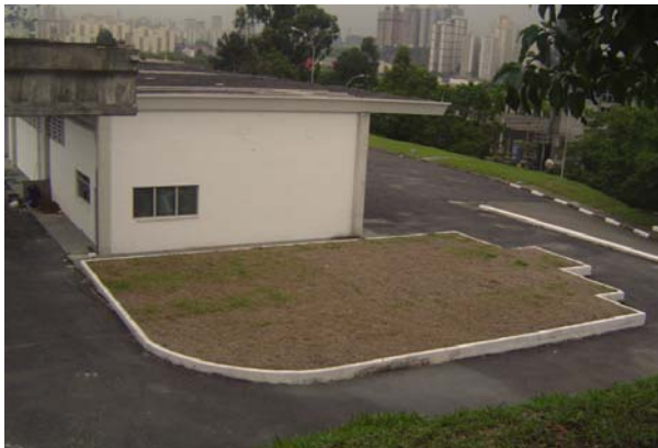
Fig 6 – Plant after D&D
