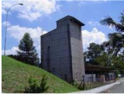
Fig 2. Pilot Plant Building
