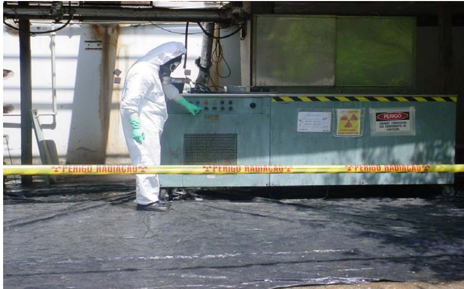
Figure 3: Signaling and isolation of areas
