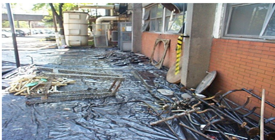
Figure 2: Signaling and isolation of areas
