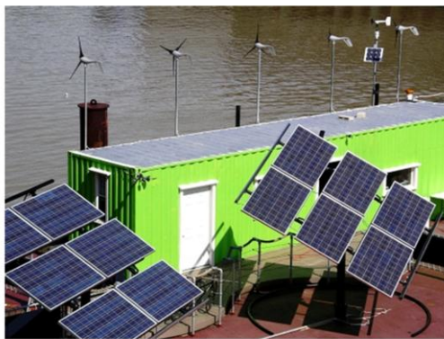
Detailed view of The Science Barge, showing the solar panels and small eolic turbines.
