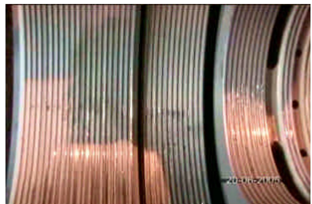
Figure 1: Damage in stationary parts
