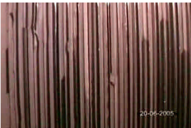
Figure 4: Damage in sealing parts
