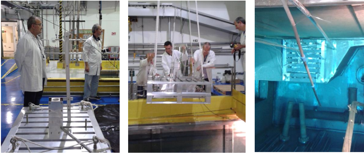
Figure 1: STAR base installation in the pool of the IEA-R1 reactor.
