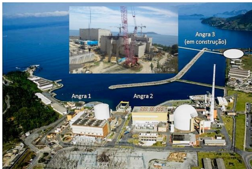
Figure 1 NPP site, Angra 1 and 2 in operation, Angra 3 buildings erection, Dec-2016
