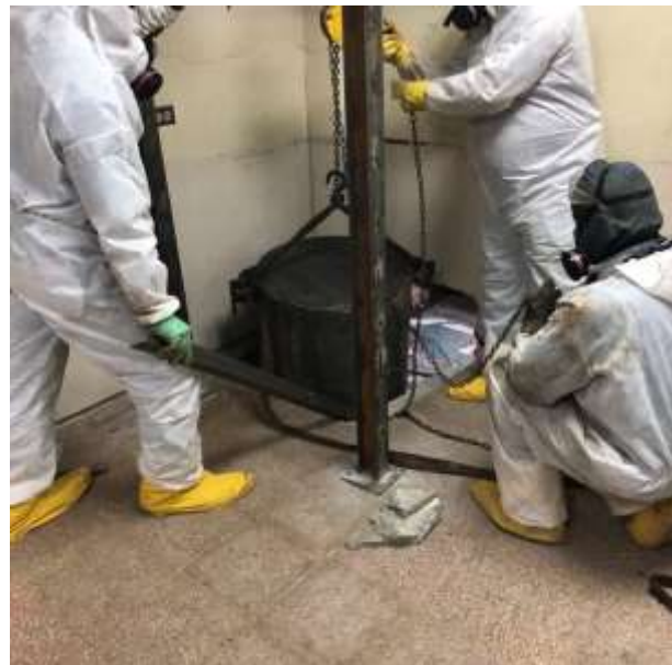
Lifting the final package
