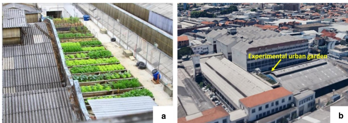
Fig. 1 a Lettuce cultivated on the rooftop and b experimental urban garden overview on the rooftop at Agronomy College
